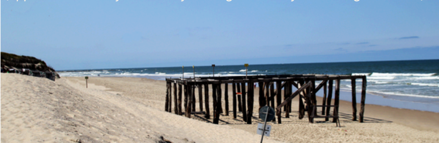
Erosion edge along the protective dune chain and former tourist platform (approx. 2 metres of sand loss following a series of storm surges in 2022)
